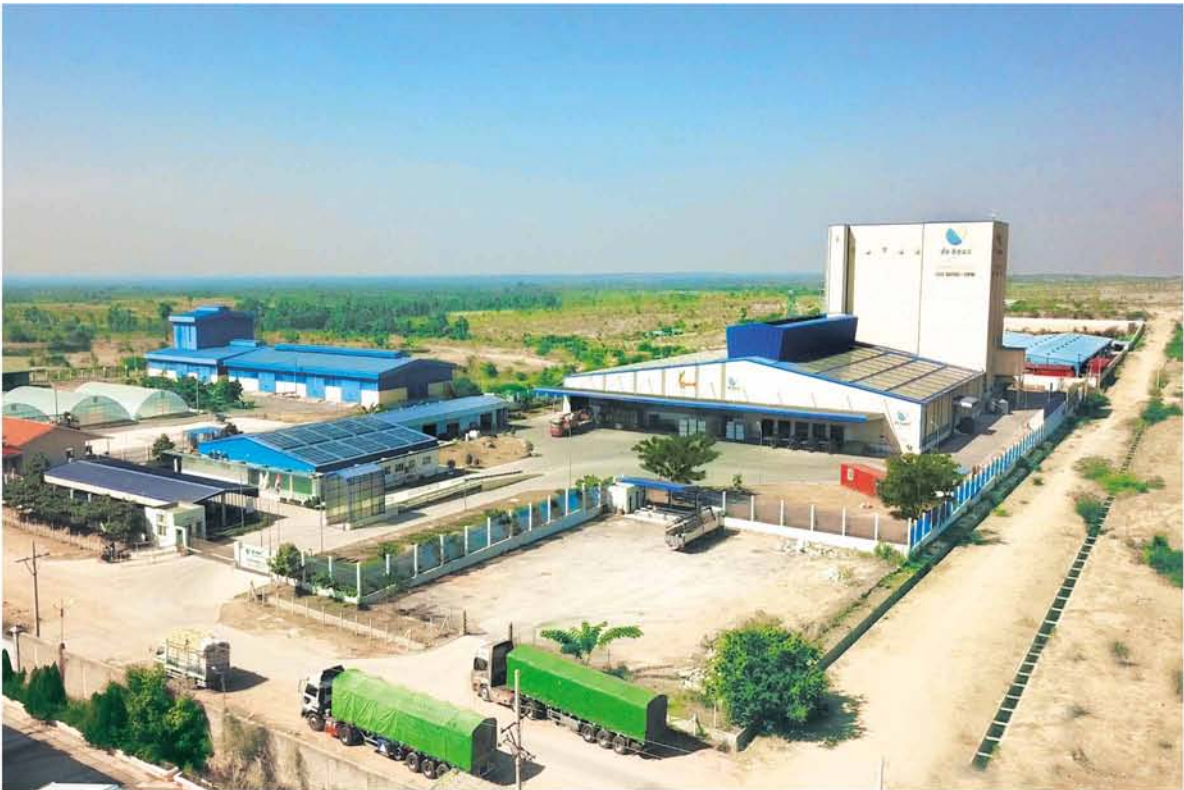
Deheus Feed Mill Factory - Netherlands
